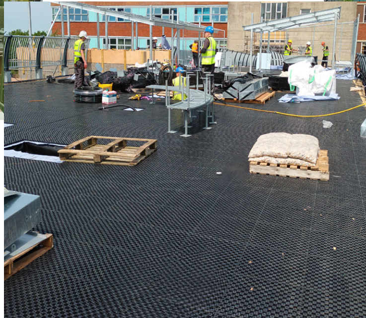
Drainage layer with attenuation and water capture.
