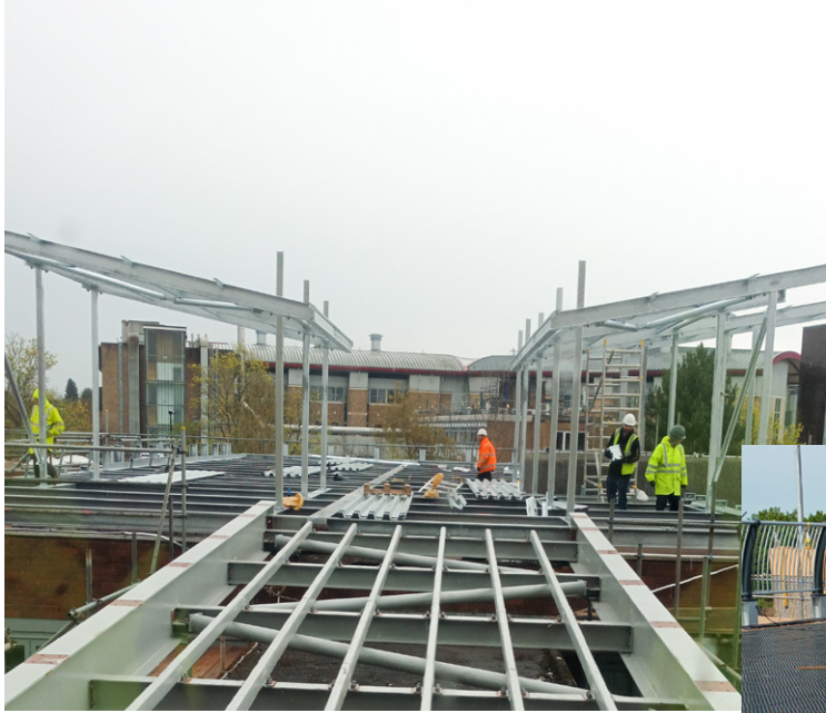
Structural frame and deck installation.
